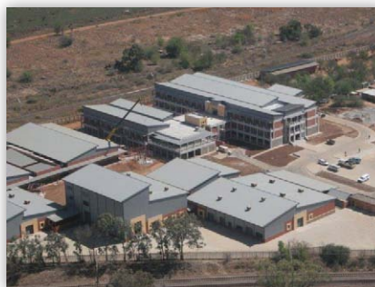
Engineering Faculty, Potchefstroom Campus
